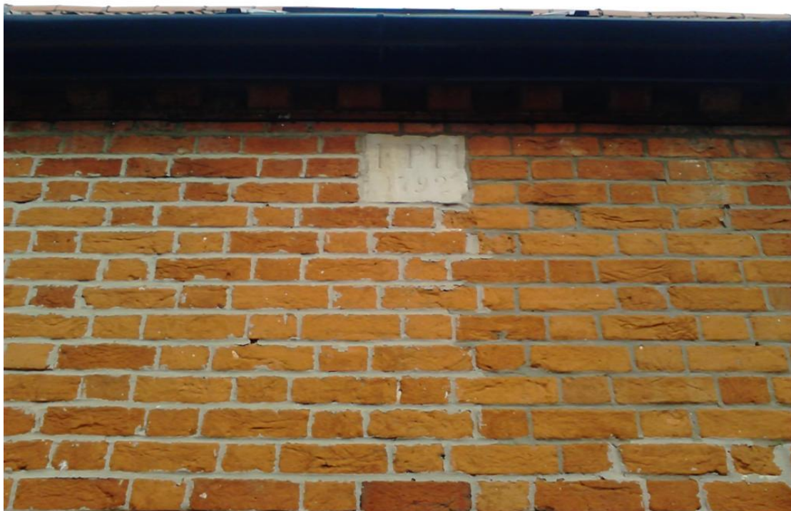
Plaque on Poor House FPH 1792
